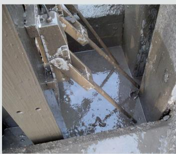
Mechanical sensors read the joint profile regardless of the width of the wall and the type of joint used.
