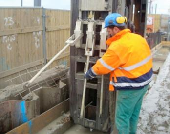
After cleaning the joint inspector with a water hose and resetting the arms, it is ready to take the next reading.
