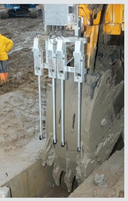
After the joint inspector is mounted to the grab unit, it scans the joint profile during one additional excavation cycle.
