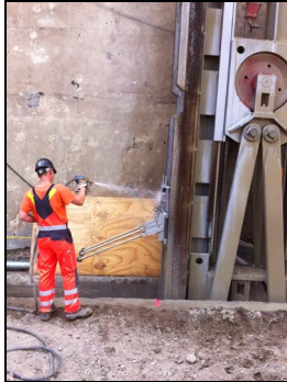
Picture 17: Test on stop end tubes
