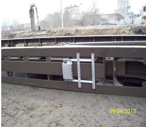
Picture 9: Modular units of the “joint inspector” without distance sensors
