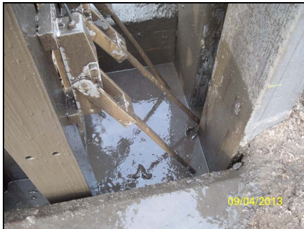
Picture 11: “Joint inspector” in touch with the joint
