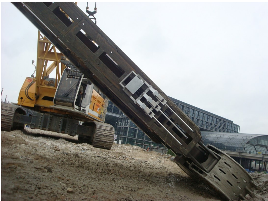
Picture 8: The “joint inspector” mounted to the grab
