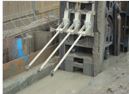
Picture 12: “Joint inspector” with fully released distance sensors
