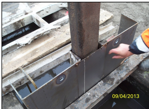
Picture 15: Test on lost stop ends
