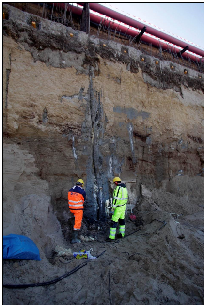
Picture 1: Repair work U2 in Berlin
