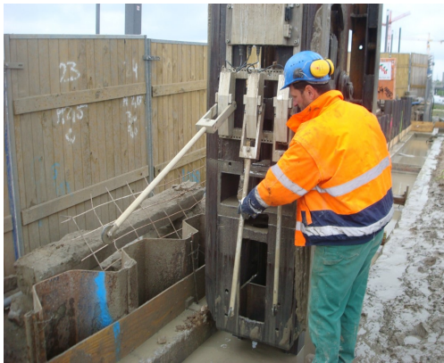
Picture 13: Test on stop ends by Bachy
